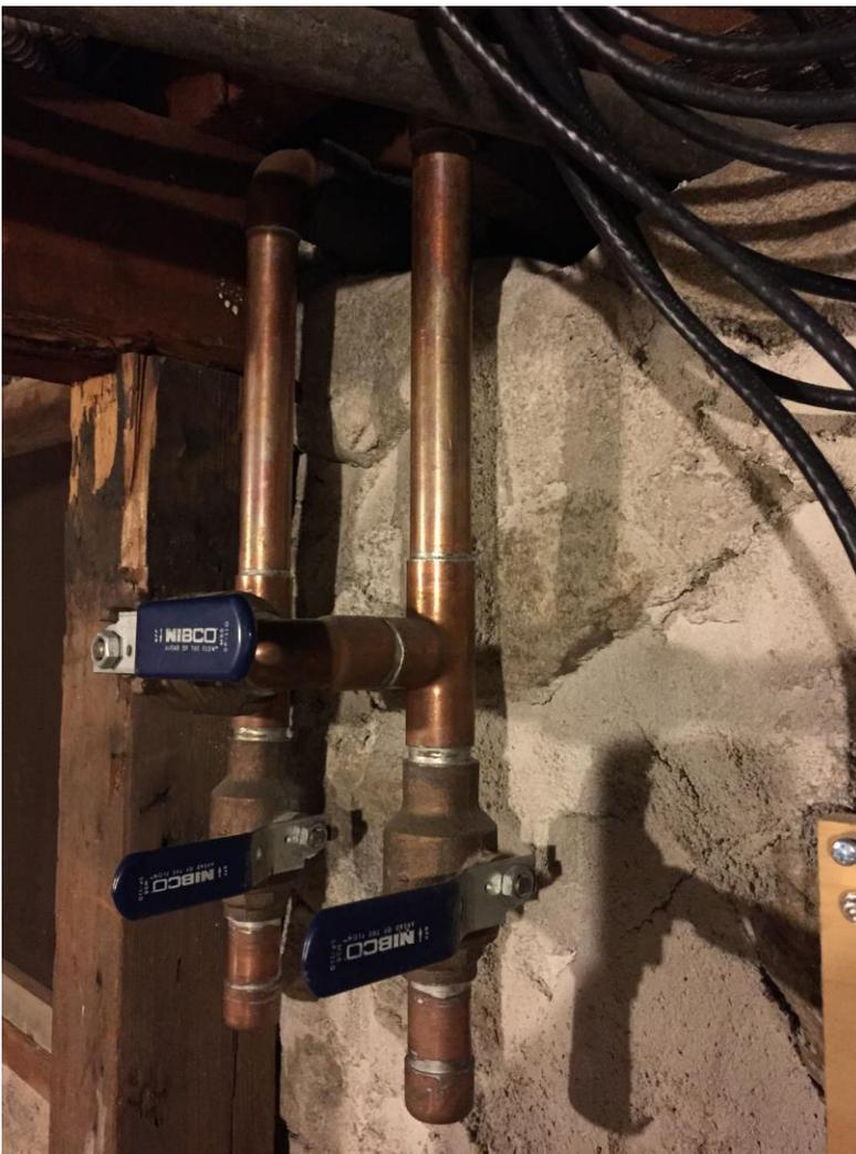
An experienced plumber should do the installation of the WaterCop. The device installs downstream of the water meter and any exterior manual shutoff valve, and is available with a valve to fit 1/2", 3/4", 1", and 1 1/4" pipes. The device should be installed indoors, such as in a crawlspace, or basement. The photo to the left shows the water line before the installation of the valve.
