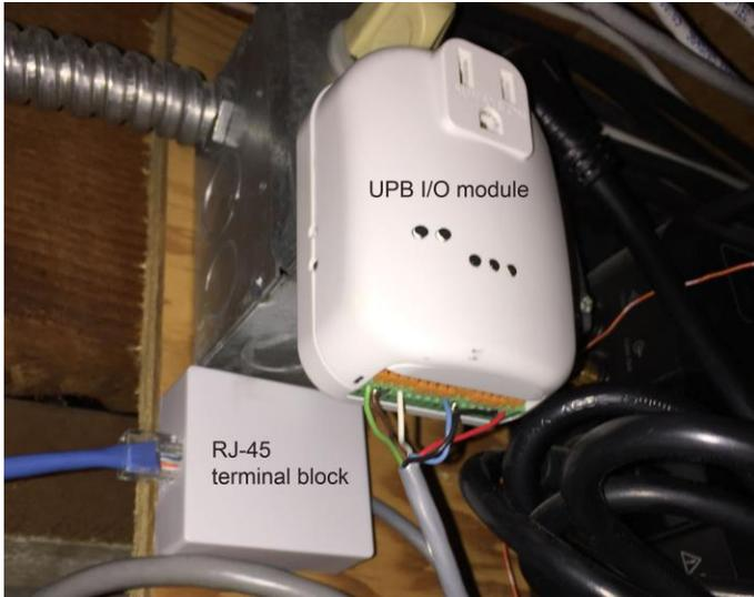
WaterCop can be integrated with HCA using a Simply Automated UPB I/O module. This module provides two momentary contact closures to open and close the valve, as well as providing two inputs that can be used to *confirm* valve opening and closing.
